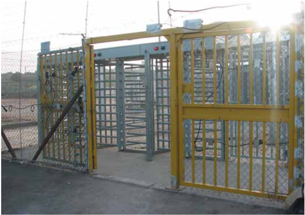
The second gate of pre-screening before entering the terminal building at Einab
